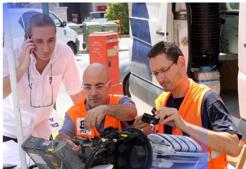
Bezeq technicians installing fiber
