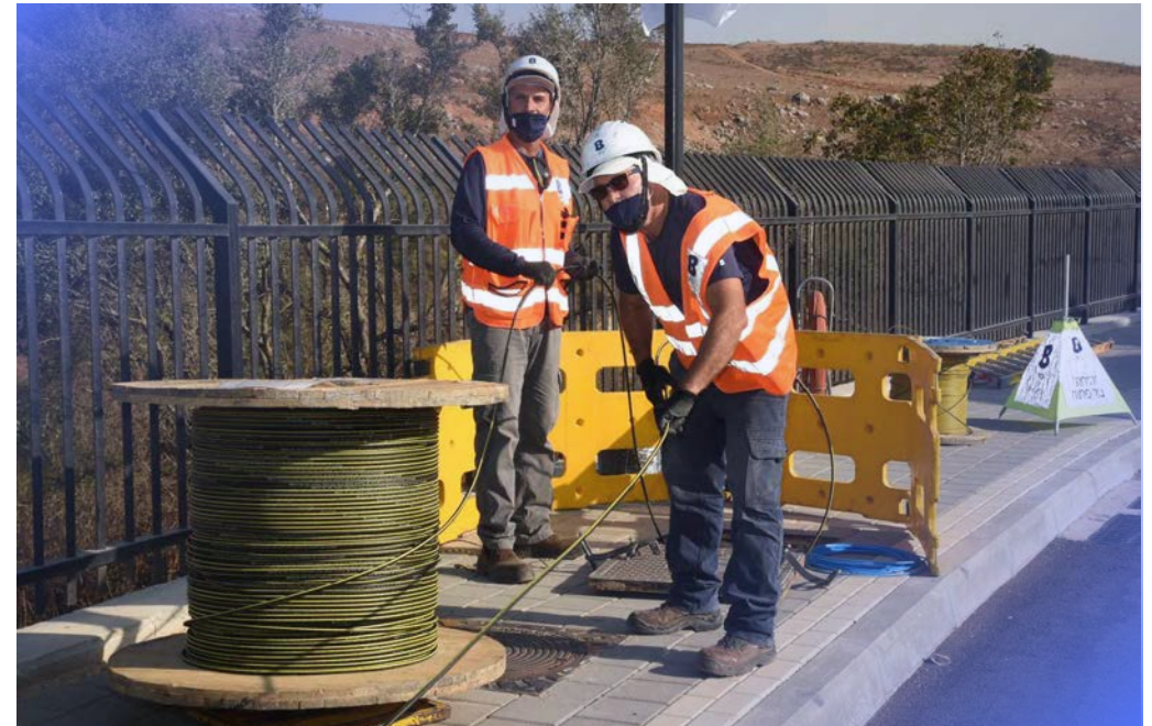
Bezeq employees deploy the fiber optic infrastructure
